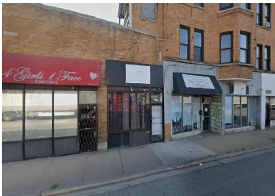
Figure 2.1. West Garfield Park Site
