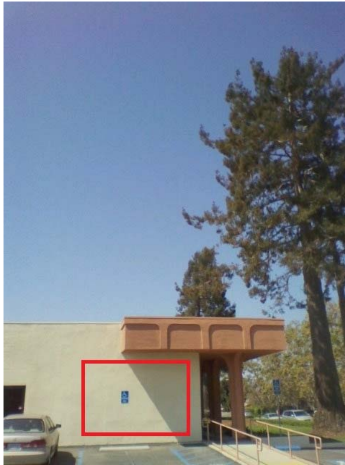
Figure 17 Exterior photo view of test room wall
