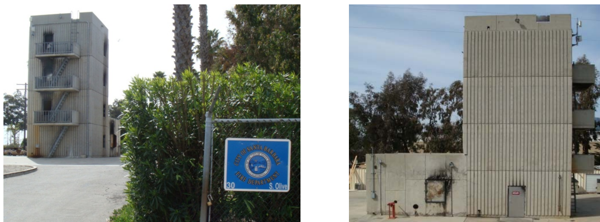
Figure 15 City of Santa Barbara Fire Tower Training Facilities
