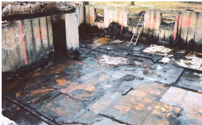
Figure II-19. Basement of structure after excavation was completed.
