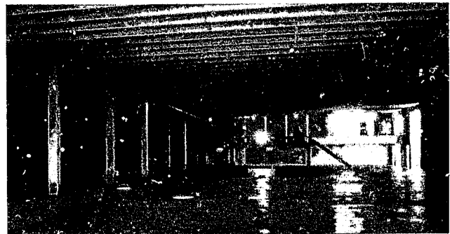
Fig. 3 Long-span double tee framing system.
