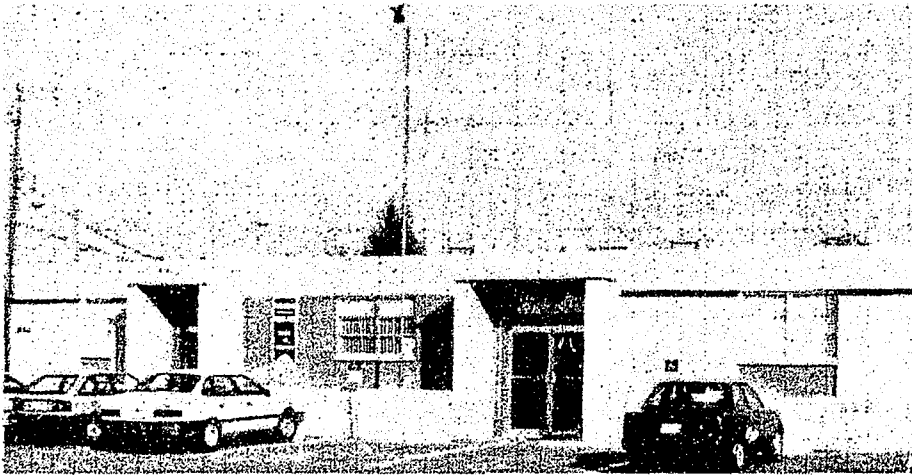
Figure 13.9 DACCO Administrative Headquarters
