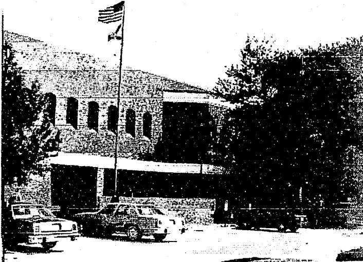
Figure 13.5 Sheriff's Office Operations Center
