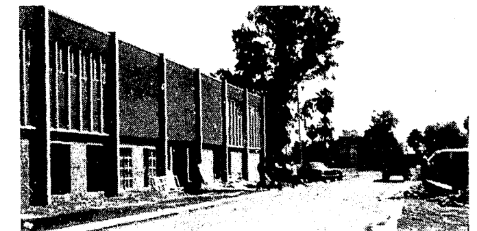
Aspen DWI Center under construction.
