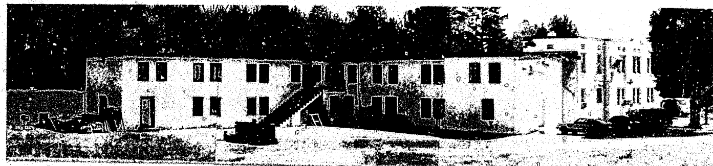
Grove Hill Community-Based Facility.
