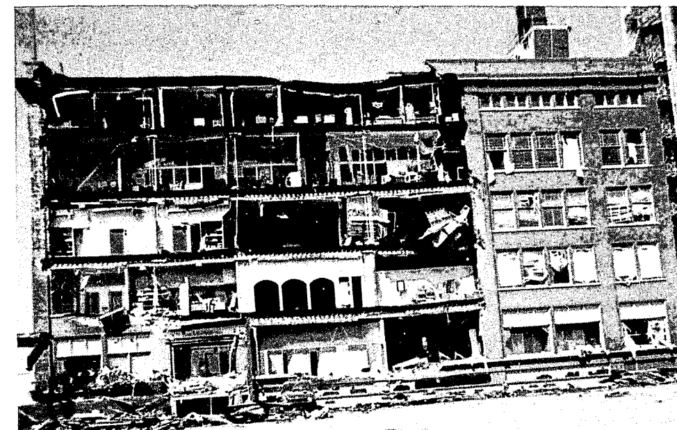
Evidence of the severity of damage caused by the May 13 tornado which caused five deaths in southwestern Lower Michigan is graphically portrayed by this photo of Gilmore's Department Store in Kalamazoo.
