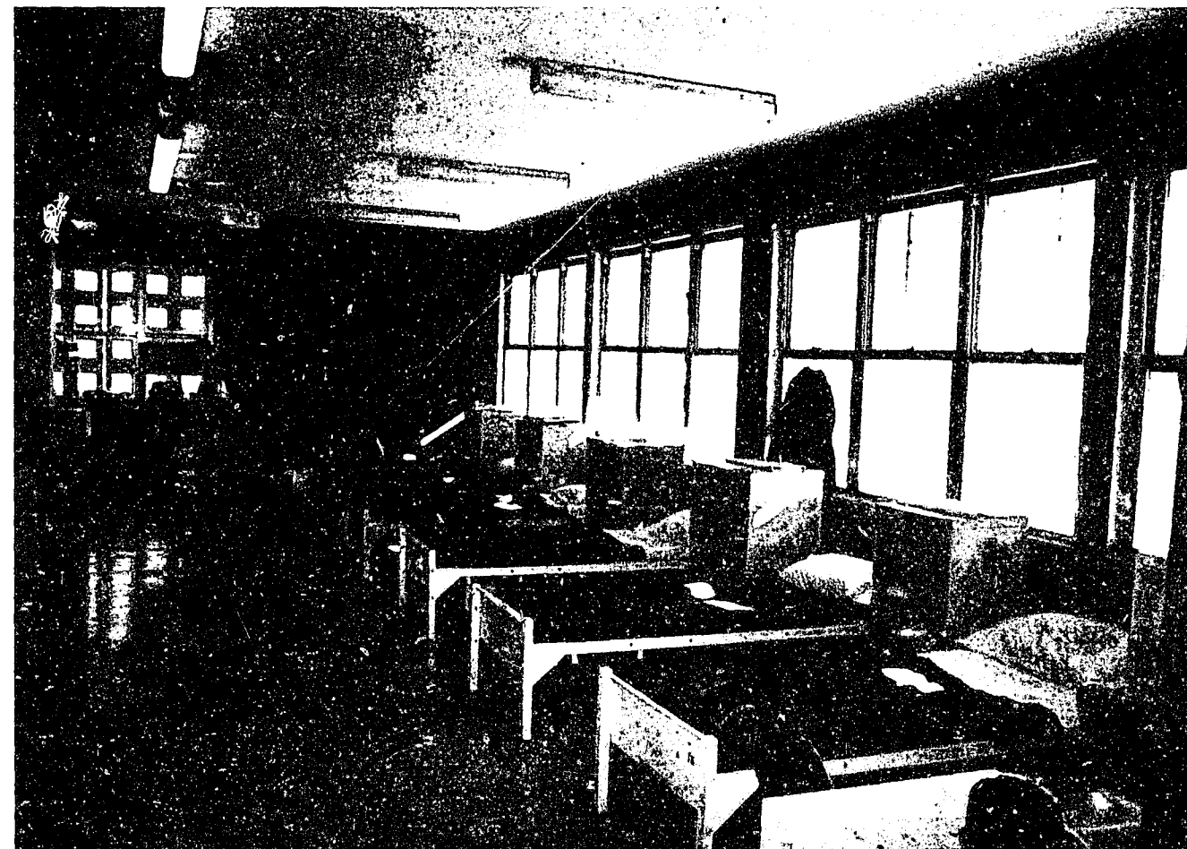
FIGURE 18. A bay of a special dormitory Texarkana Federal Correctional Institution.
