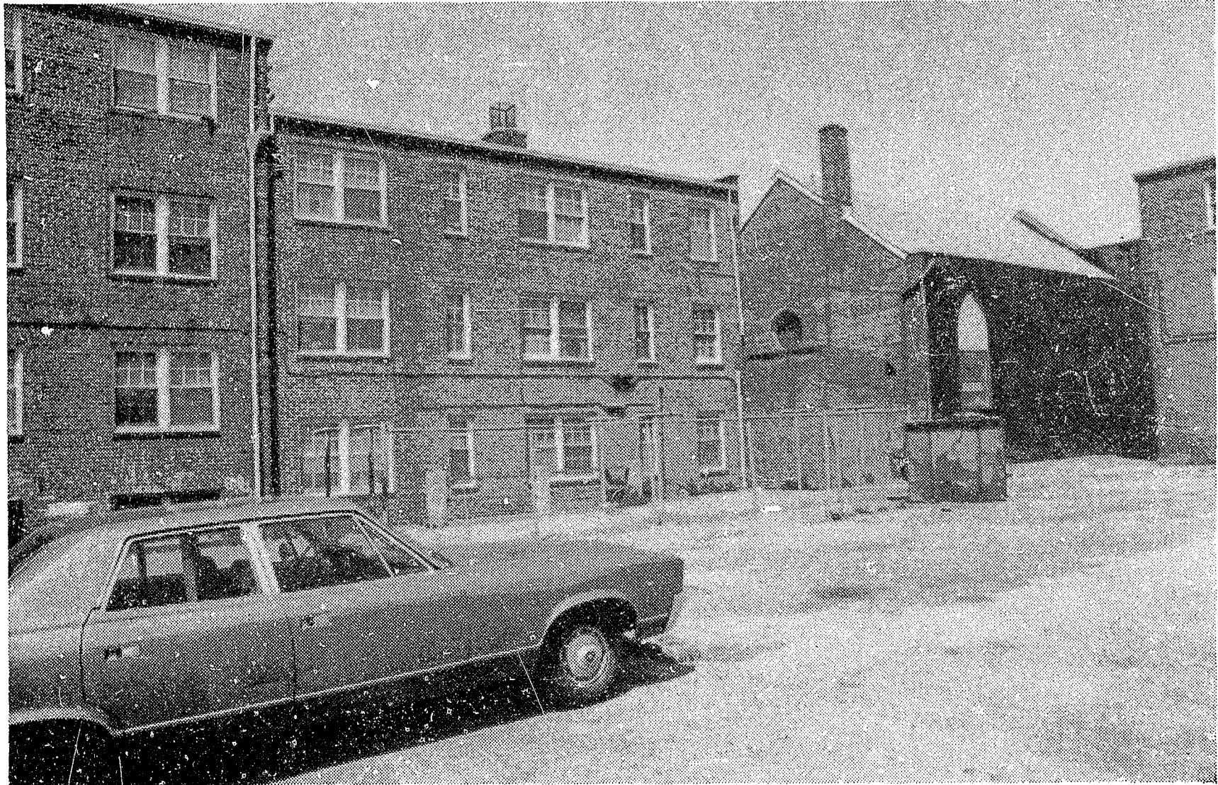
Figure 16: Photo: Carrollsburg Rear Yard Area Rear yard areas in Carrollsburg are undifferentiated and poorly used
