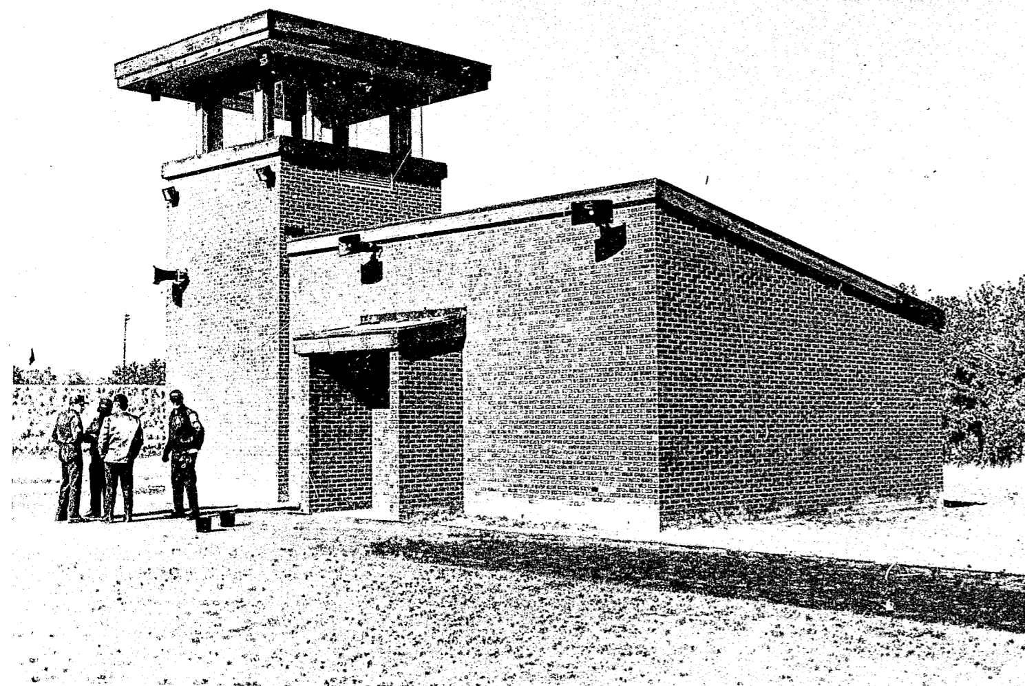
Range tower and storage building.
