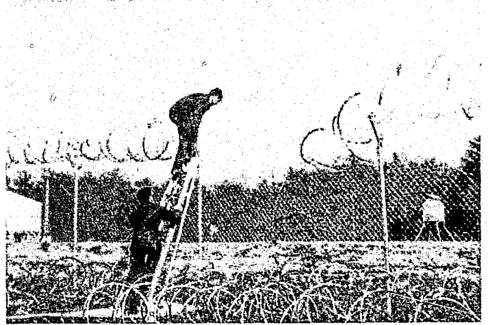
FIGURE 10. Fence Array No. 25.
