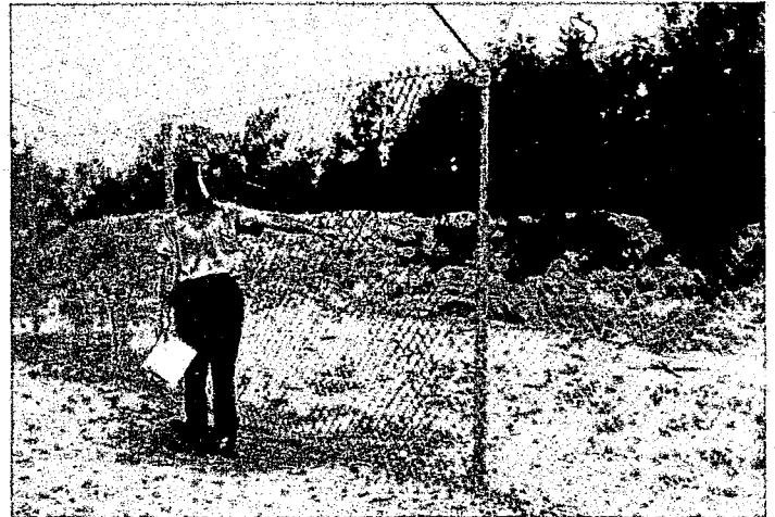
FIGURE 12. Damage caused by rocket attack.
