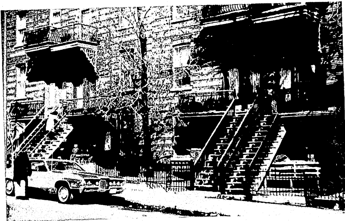
Figure 2.12: Walk-up flats in Montreal, built at 50 units to the acre. All entries face onto the street; there are no interior public spaces.
