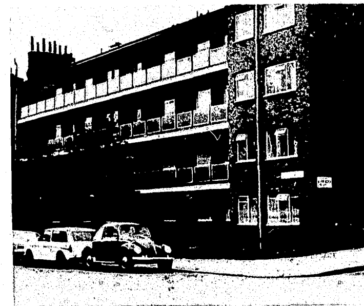
Figure 2.14: Example of a four-story walk-up in London. Each apartment is on only one level, and all entries are off single-loaded corridors facing the street.
