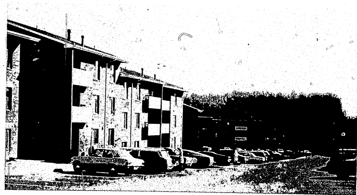
Figure 2.11: Contemporary suburban garden apartment, or walk-up, built at 35 units to the acre.
