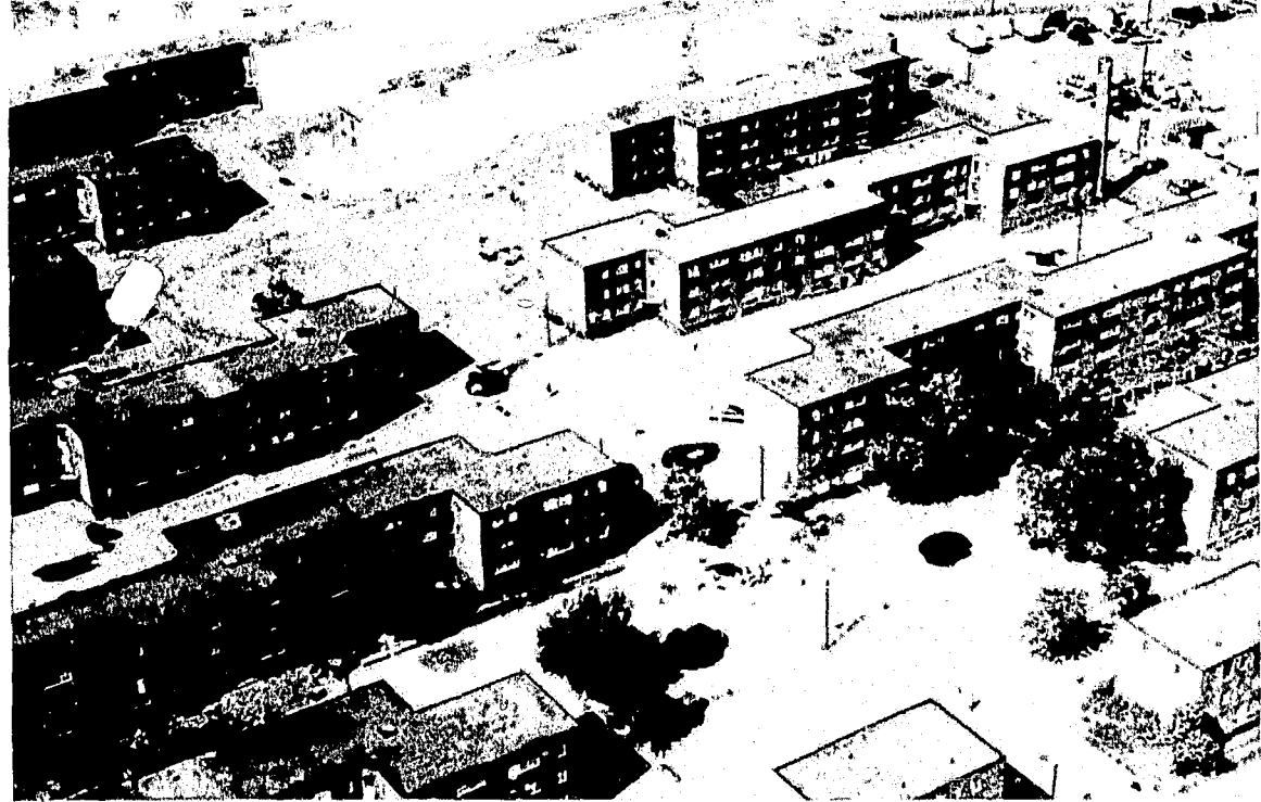
Figure 4.5: Aerial view of a housing project, showing the virtual wall-to-wall asphalted of the grounds area.
