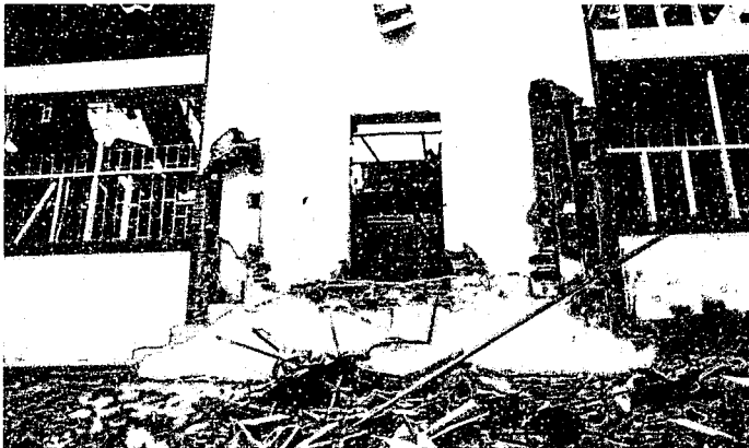
January 23, 1994—Bucaramanga, Colombia: Damage to a Mormon chapel in Bucaramanga caused by a bomb planted by suspected Marxist guerrillas.
