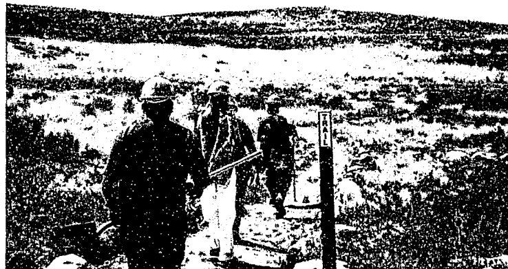
Work crew on site at Antelope Island.
