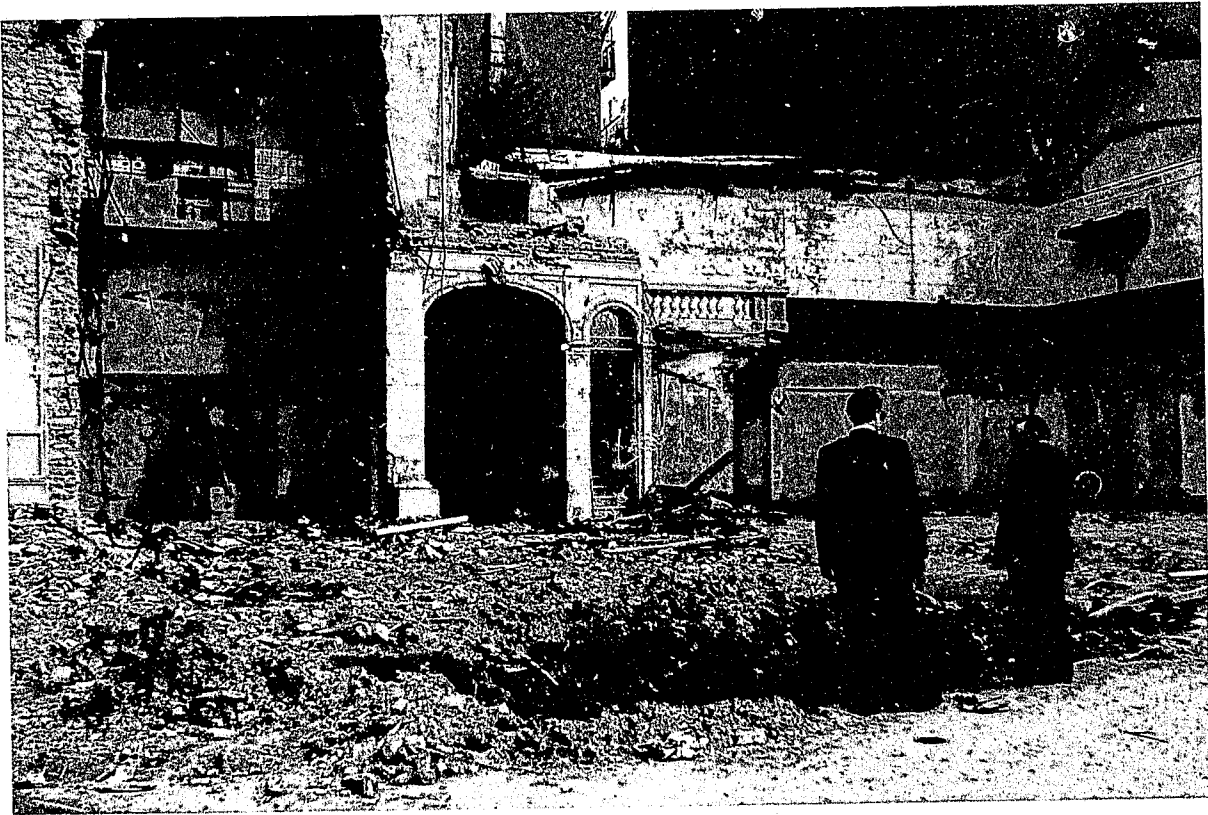
Blast seat of a large vehicle bomb and the resultant damage to the Israeli Embassy in Argentina.
