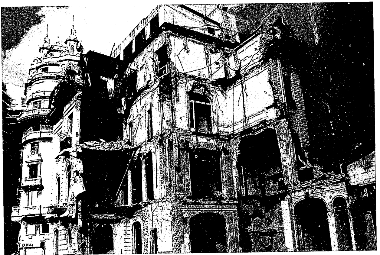
Blast seat of a large vehicle bomb and the resultant damage to the Israeli Embassy in Argentina.
