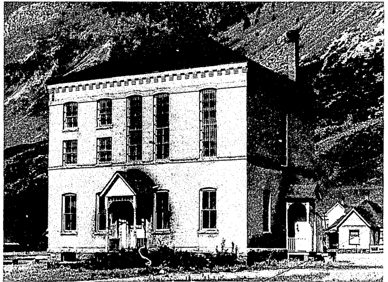
Silvertown, Colo., Jail. (Ca. 1930)
