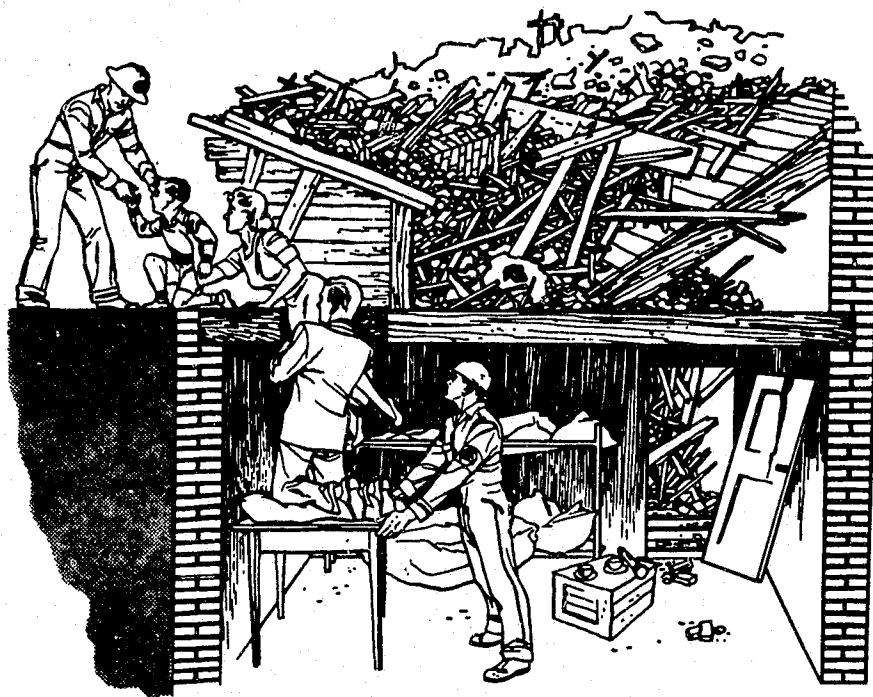
FIGURE 58.—Tunneling to gain entrance.
