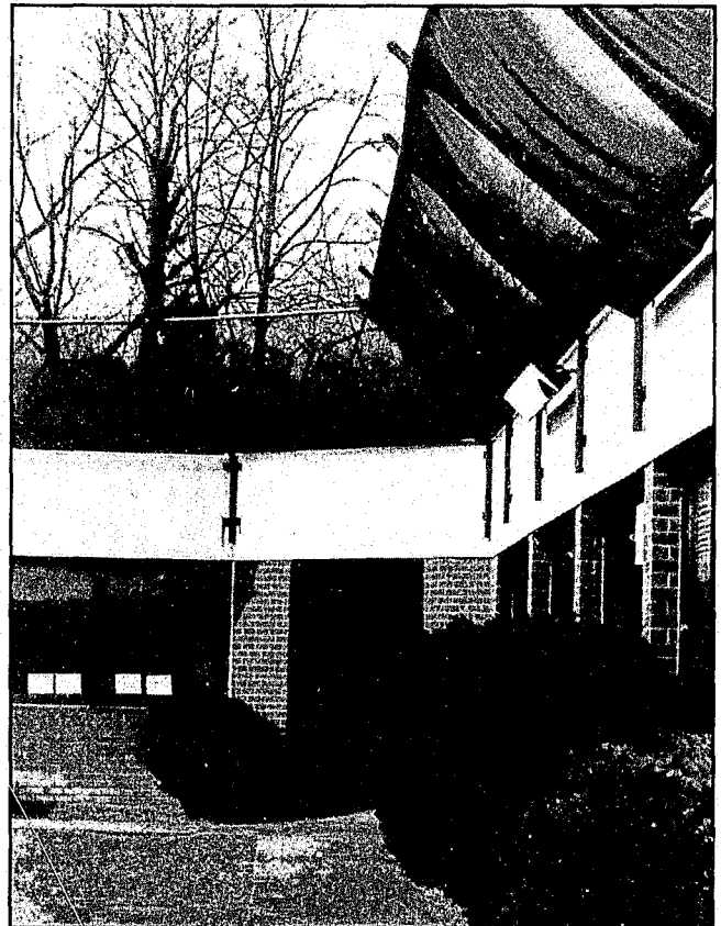
Inside Courtyard Fence
