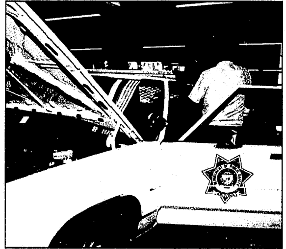
Light bar installation.
