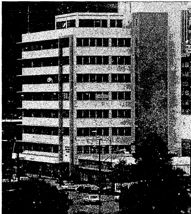
SALT LAKE CITY PUBLIC SAFETY BUILDING
