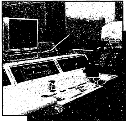
Top right: Windows into the Emergency Operating Center are on the left, the Observation Gallery on the right and the CAD computer is pictured lower left. Bottom right: A typical 9-1-1 operator console—there are 10 of these—features an adjustable keyboard shelf and a low console profile.
