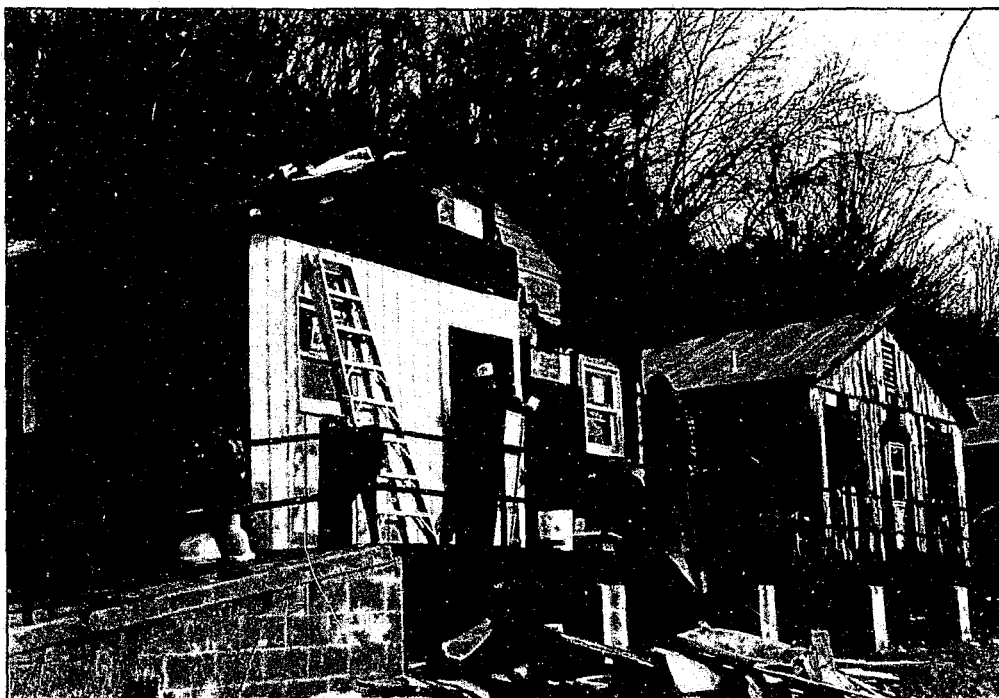
Participants in the State Intensive Supervision Program are renovating cabins at Voorhees State Park for use by the Department of Corrections as a residential treatment center for juvenile alcoholics. (Photo courtesy of the State Intensive Supervision Program.)
