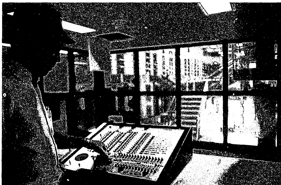
A construction worker inspects electronic controls for a cellhouse at the new Danville Correctional Center, opened in October 1985. The Danville prison is similar in design to the Henry C. Hill Correctional Center under construction at Galesburg and the Shawnee Correctional Center in Vienna. Cell doors are all controlled from one central room, reducing the number of security personnel necessary.
