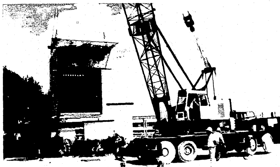
A crane lifts one of the innovative cell modules into place at the Florida Mining and Minerals Plant in Tampa, Florida.
